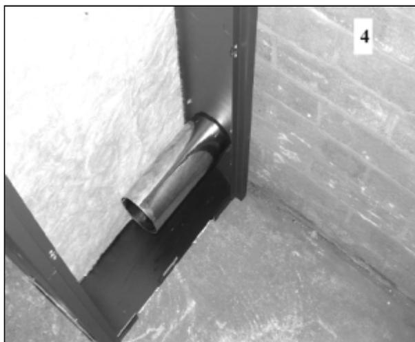
It is possible to route the flow and return pipes through the back panel. To do this you have to remove the door lock and move the complete lock assembly to the opposite end of the door. Invert the door assembly and fix the duct seal and plate using the nuts and washers provided. Make sure the plastic blanking cap is fitted to the hole vacated by the lock assembly.
