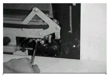
Cut a cross slit in the rubber grommet and feed the appliance onto the 8mm-gas supply pipe. Position the restrictor elbow supplied and mark supply pipe at its cut off length. Remove appliance, cut pipe to correct length, refit appliance and make gas connection with restrictor elbow use 15mm A/F spanner taking care not to apply any force to the gas control spindle as above. Ensure the restrictor valve is opened and its cap replaced tightly.
