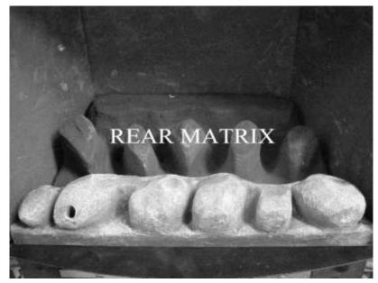
Position the front row of "A" & "B" shape pebbles as shown.
