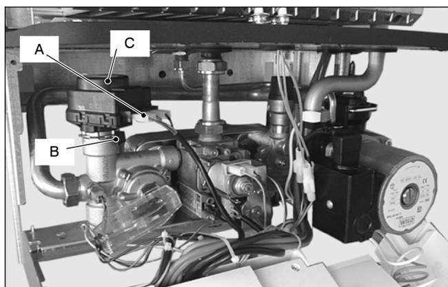
**64 DIVERTER VALVE INTERNAL PARTS REPLACEMENT**
