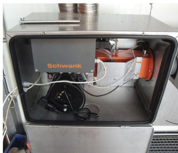
Fig. 63: Mounted burner kit in protection cover with gas inlet and electrical connections
