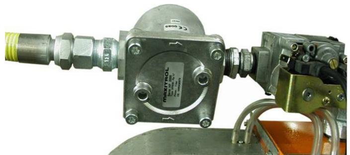
Fig. 61: Mounted gas filter group at tube heater
