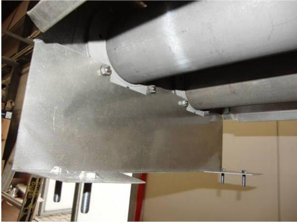
Fig. 50: Fixed end bracket on turnaround box
