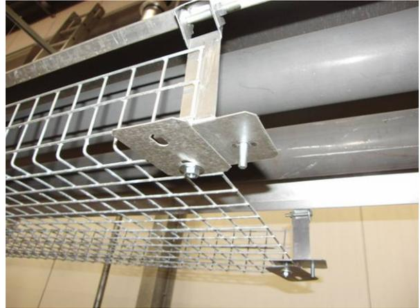
Fig. 53: Loose mounted clamp
